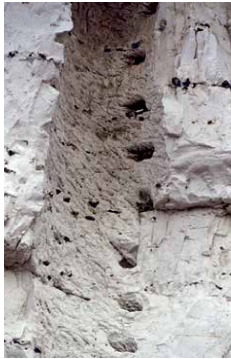
The Belle Tout shaft as exposed in the 1970s, with the shaft and its fill (left), and foot holes (right) (Photos: David Freke 1976).
