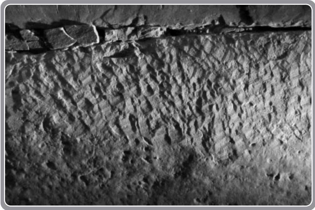
Chisel working at the top of the large stone at the base of the north buttress, Maes Howe
